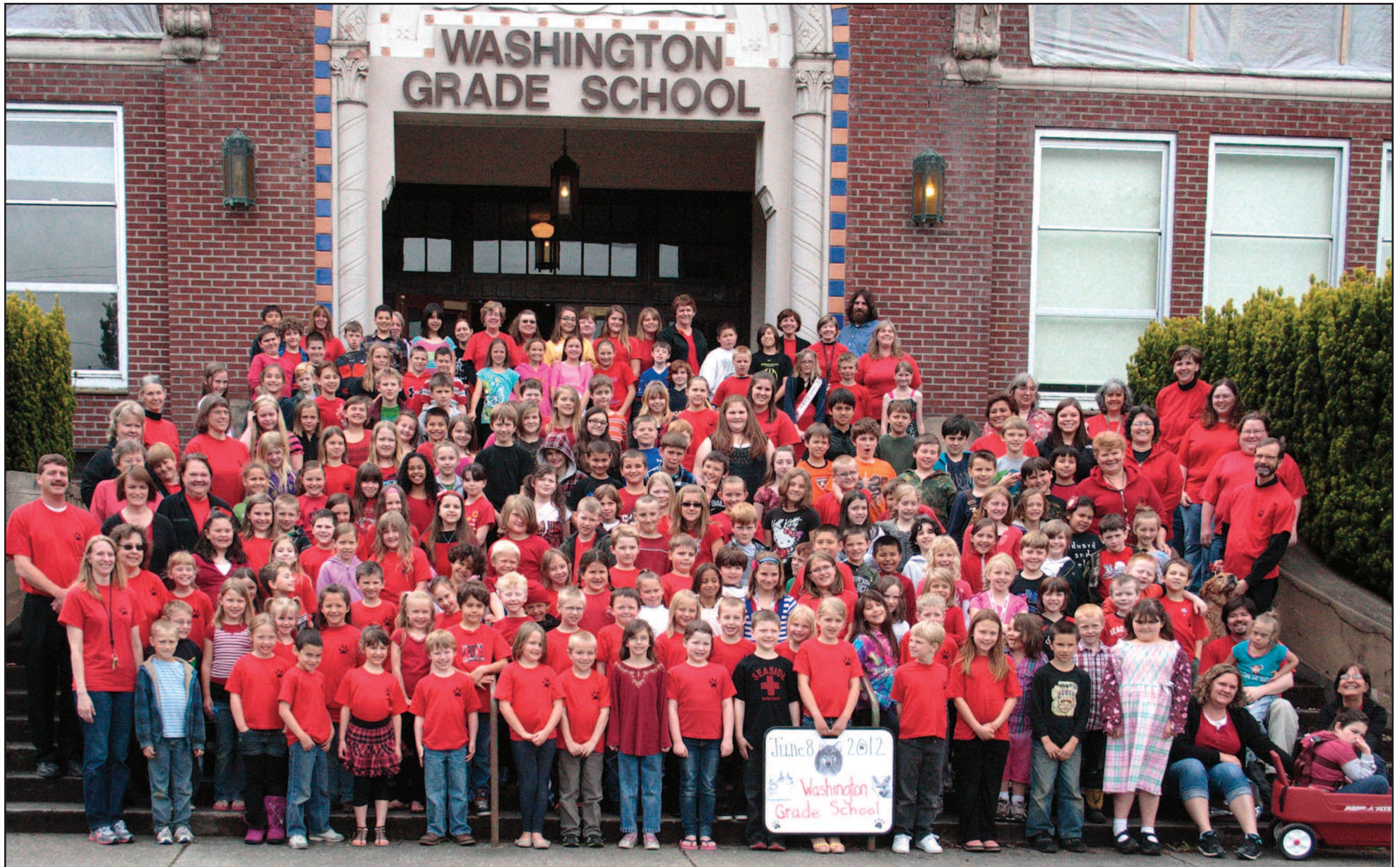
On June 8, the staff and students of Washington Grade School were encouraged to wear red and black for this final picture in front of the school. The school will be demolished starting in July and classes in September will be held in the new school building on Missouri Ave. The new building will house Kindergarten through 12th grades. Photo by Clark McGaugh
