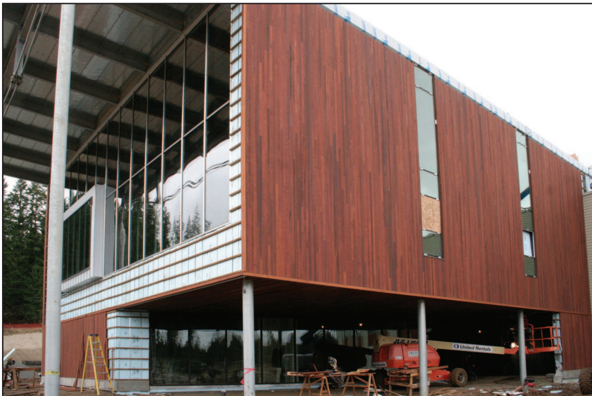
The new Vernonia school building continues to take shape. This picture, taken January 31, of the front entrance shows many of the windows in place and FSC cedar siding. The FSC designation assures that the wood was responsibly harvested from well-managed verified sources. For more information on the new school and funding, see article on page 12 by Superintendent Dr. Ken Cox.
