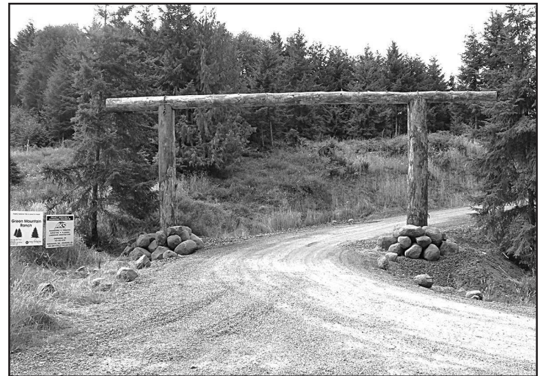
The entrance to Green Mountain Ranch Oregon is framed by log posts, made from trees cut on the property, that are 2.5 feet in diameter and 20 feet tall, and topped by a 1.5 foot diameter log.
