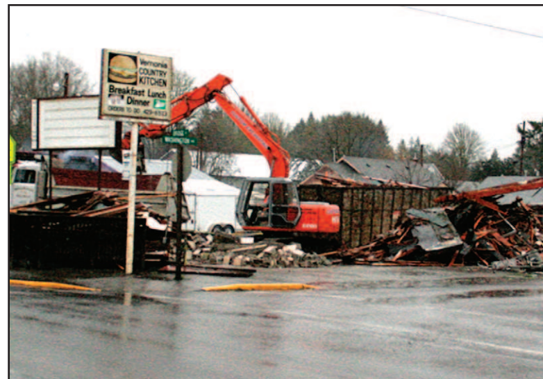
February, 2011, demolition crew carefully dismantles café.
