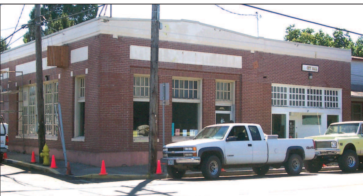
Banks City Hall shown at the beginning of the renovation on the building, was built in the 1930s as a bank.
