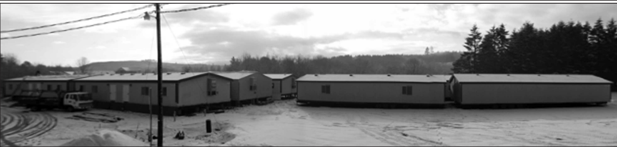
The new temporary modular buildings are being put in place behind Washington Grade School as weather allows. This picture was taken on January 15 after snow fell overnight.
