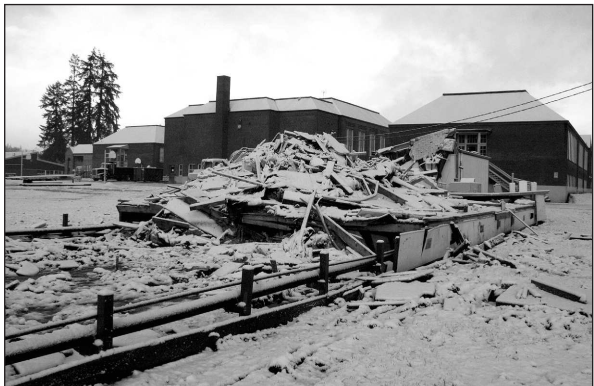
The old modular building behind Washington Grade School being demolished to make room for approximately 3,500 cubic yards of gravel needed to level the area around the old building in preparation for new temporary modular buildings that need to be in place before school can start back up in Vernonia.
