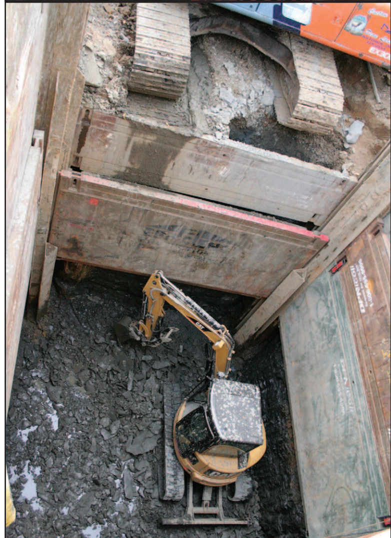
Pictures above and left show excavations on waste water pump station 2. The new wet well is scheduled to be completed this week as part of Phase I of the city's waste water improvements.
