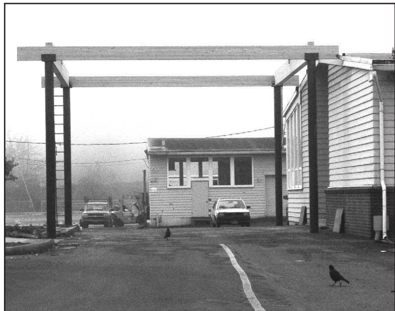
Above, work is in progress to replace the portico beside Vernonia High School.
