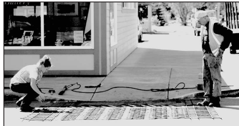
Above, employees of BRIX, a company hired by the State of Oregon to construct crosswalks, place the stamp template in the crosswalk after using an infrared heater to warm up the surface so the stamp will imprint. After the surface cools, four coats of a cementitious color coating is applied.
