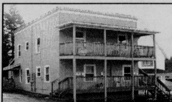
GREAT INVESTMENT OPPORTUNITY! Almost NEW 6-Unit Apartment Complex in downtown Vernonia. Remodeled in 2000. $279,000 Call Patty 503-704-1381
