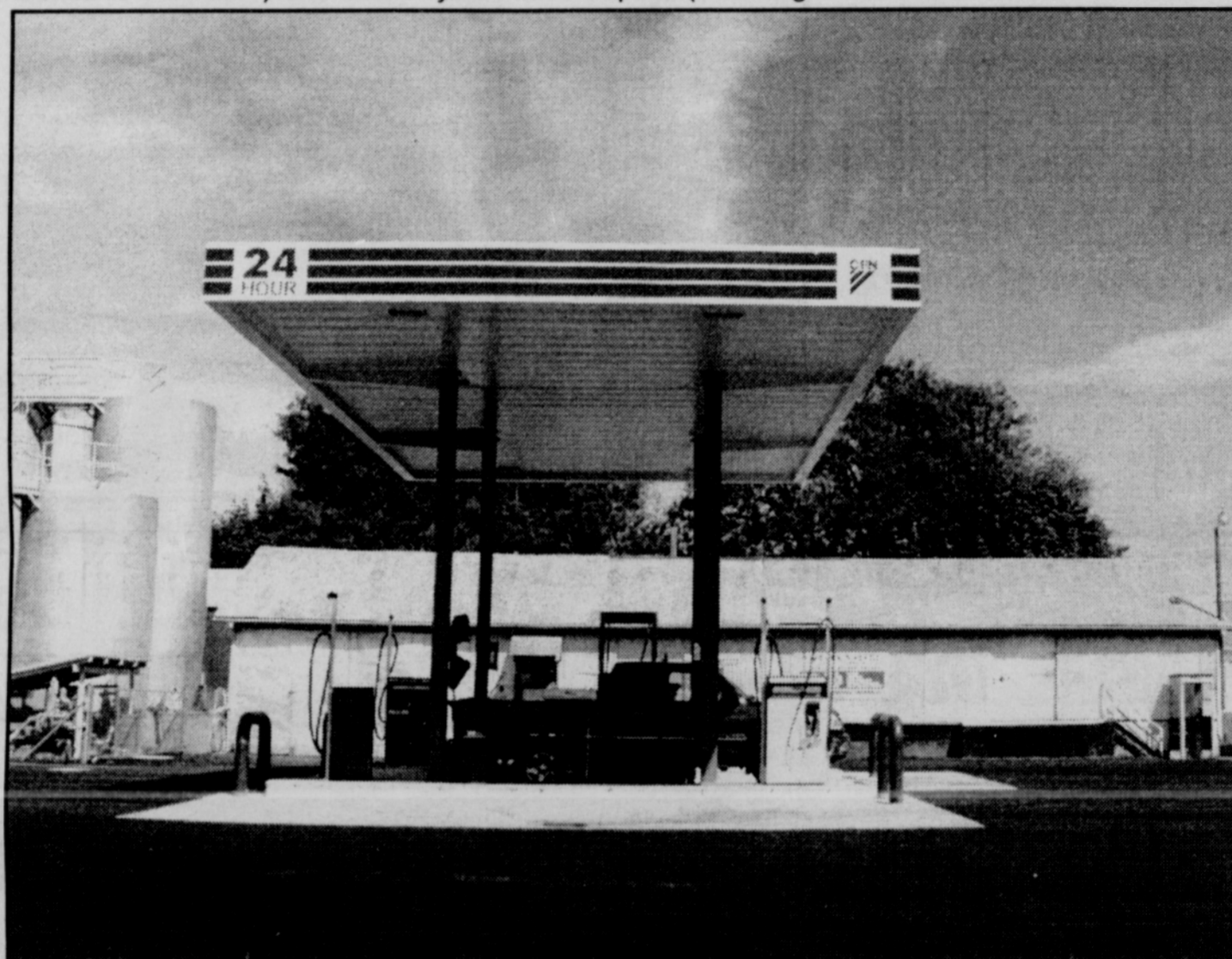
New service islands, modern piping and a paved street make the Wilcox & Flegel cardlock in Vernonia more pleasant and convenient than ever.
