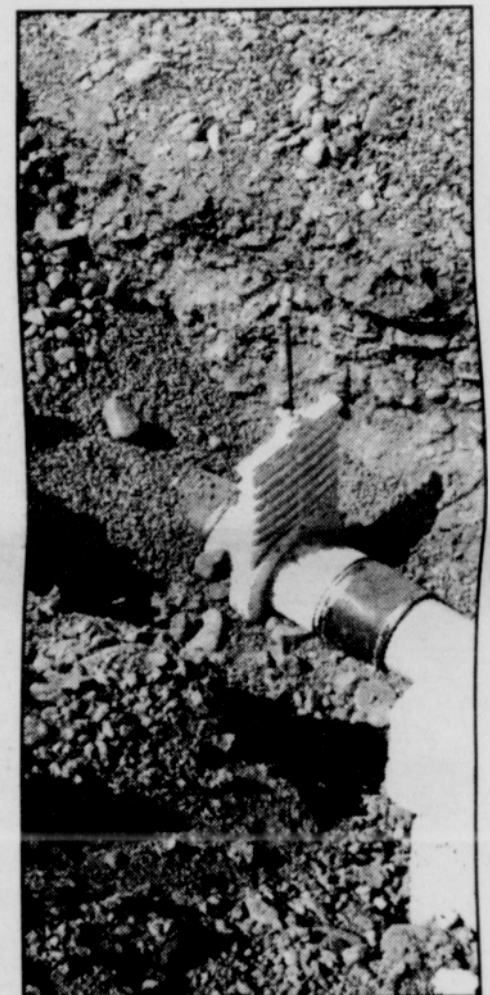
This simple-looking combination of plastic and metal is a key element for containing a fuel spill, or for shutting off the flow of fuel in case of fire.
