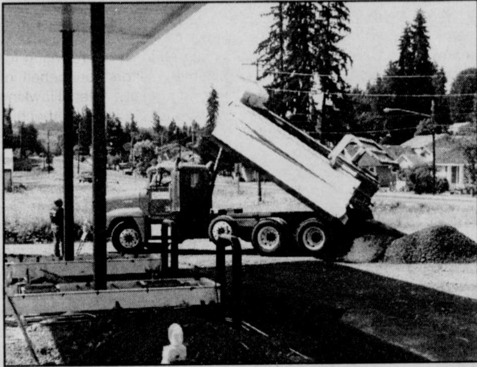
Two more loads of gravel arrive from Morse Bros. Deer Island facility.
