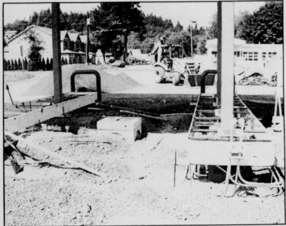
Pipes and sumps are visible during construction of Wilcox & Flegel's new cardlock.
