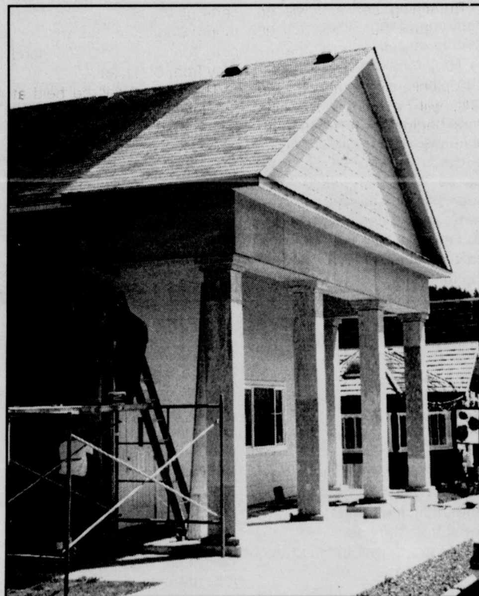
Paul Pastor Jr. and Del Allen (on ladder) at work on the new front of the Vernonia Foursquare Church. The congregation has been steadily improving their facility, starting with a new sidewalk last year, then remodeling and extending the front to create space for a new church office. The roofed front entrance and pillars create an inviting structure.
