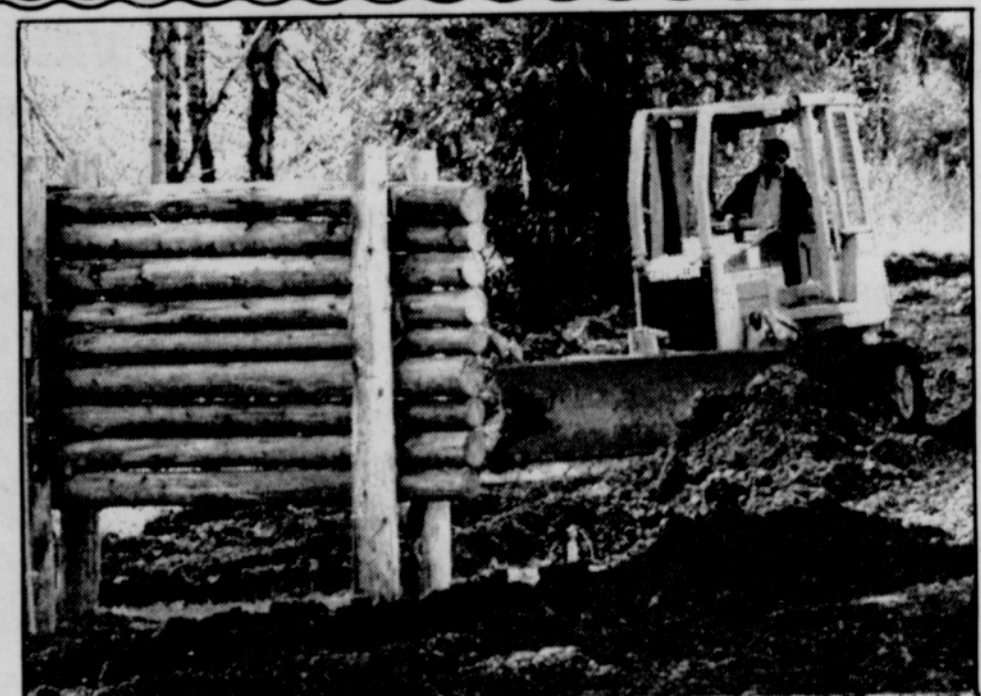
A lot of fill and grading was needed at the entrance to town, where a trail was also added from Hwy. 47 to the Linear Trail.
