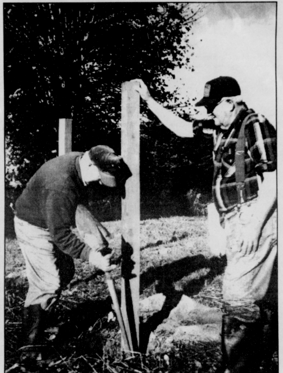
Ralph Keasey, left, installed new fence posts at Pioneer Cemetery with the aid of Ben Goodman and other members of the LDS Church congregation.
