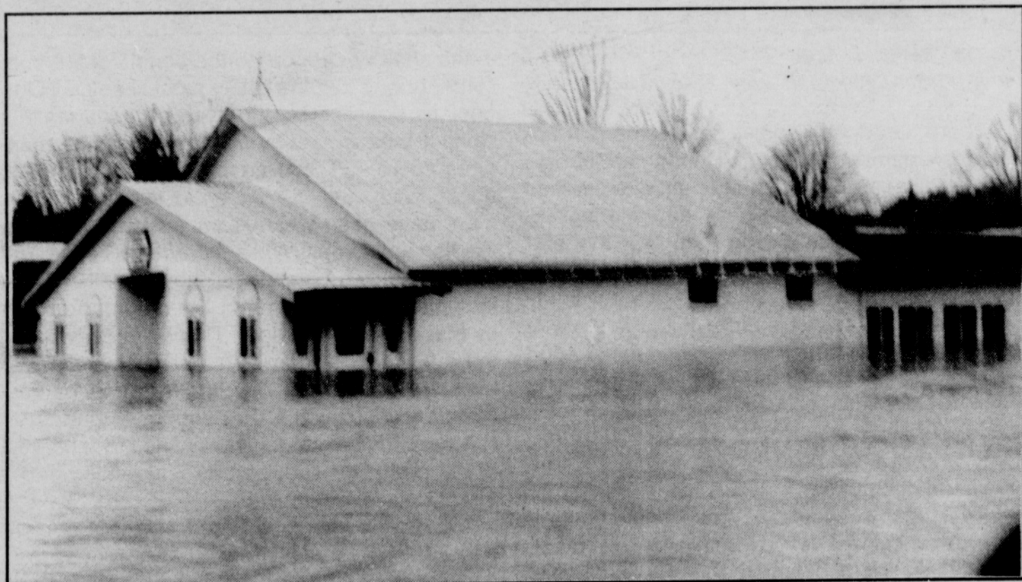
This photo is of the Vernonia Senior Citizens Center before the flood crested, forcing nearly four feet of water into the building.
