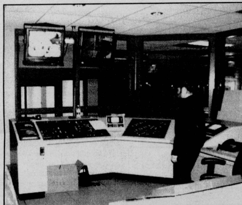
Nerve center for the new facility is this open area that allows a direct view into the cell pods, with cameras to cover areas lacking a direct view. It is designed so that one person can monitor all areas and also control all doors except the main door from the public parking lot.
