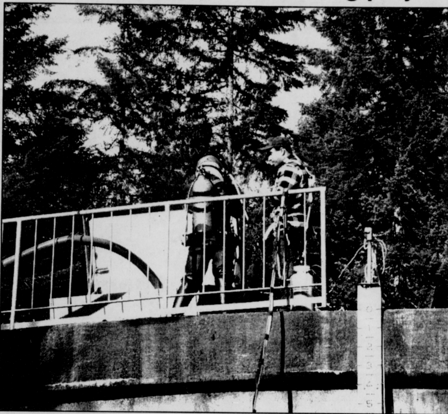
Mark Harvey, in diving gear, and Chad Masi make preparations to start an inspection of the interior of the Stoney Point reservoir. The large hose on the left is a vacuum hose that will remove sediment from the bottom of the reservoir.
