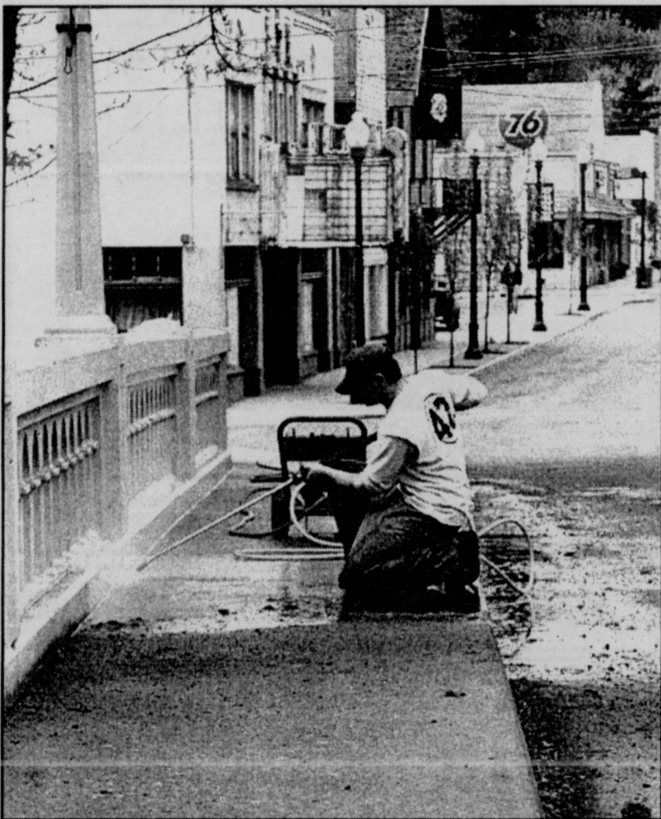
A thorough pressure washing prepared the bridge in advance.
