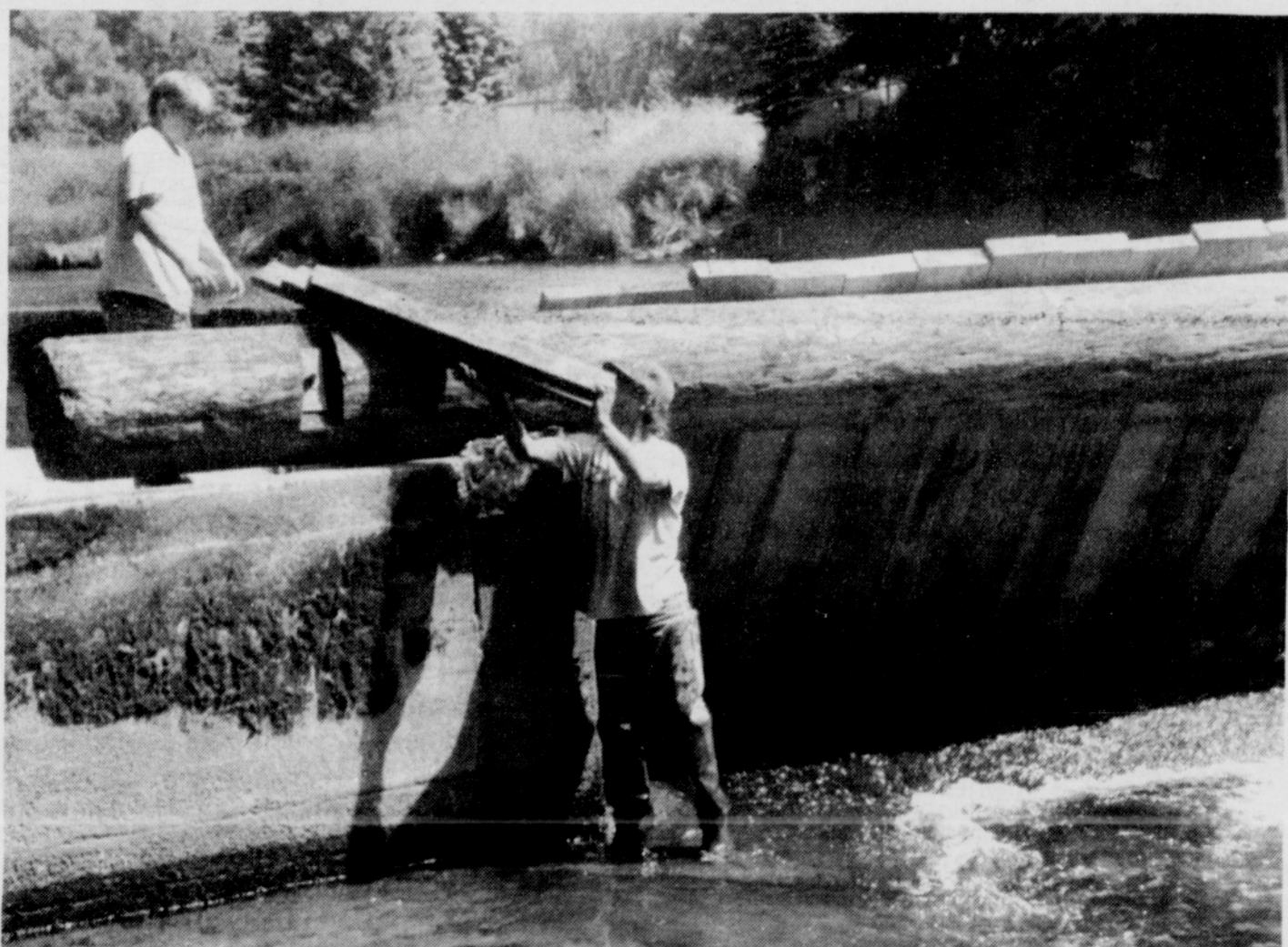
Jeff Burch and other Vernonia Public Works employees found lots of hands eagerly wanting to help install the dam on the city's Rock Creek Swimming Pool. This annual rite of summer was just in time for last week's hot weather.
