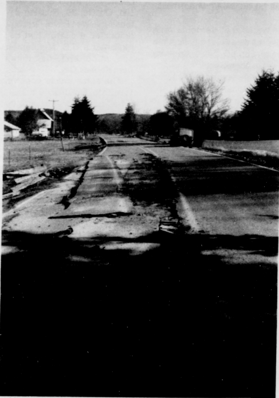
Hwy. 47 at Natal fell apart between the center stripes.
