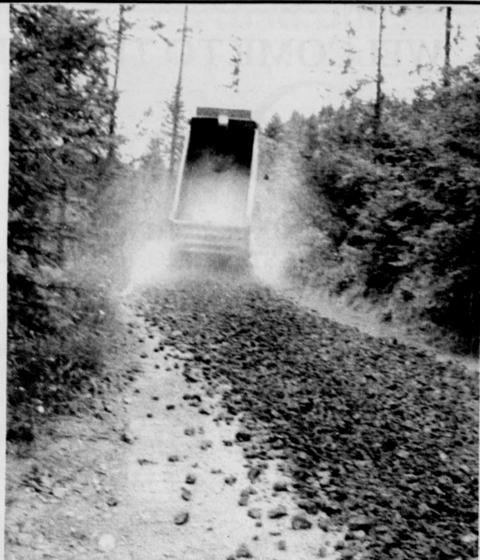
Spreading a load helps reduce the work later.
