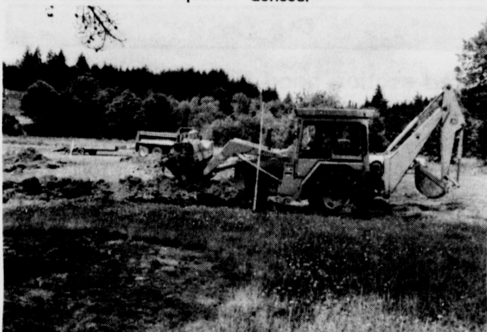
Dick Titus of Northwest Excavation prepares footings for the first home in the Cedarwood Addition of Vernonia.
