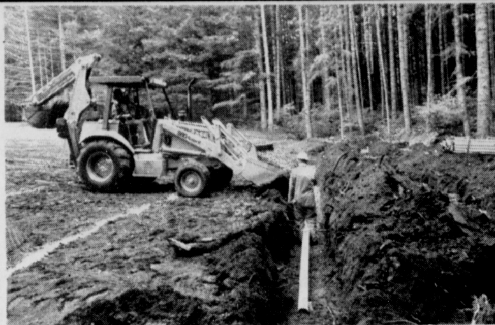
Kelly and Tim Lungberg, father and son employees of the Columbia County Road Dep't., install and cover pipe in a new drainfield at Camp Wilkerson.
