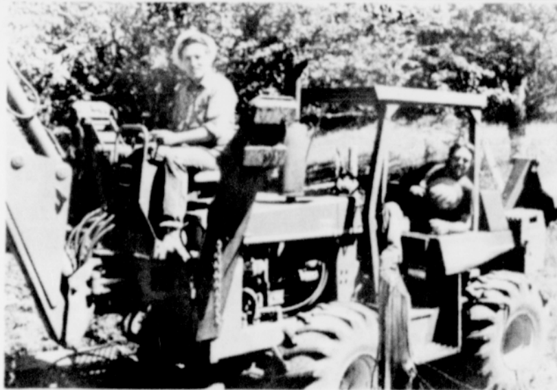
Dee, left, and Lance Stevens use their 7510 Ditchwitch horizontal boring unit to install conduit under Stoney Point Road for a new residence.
