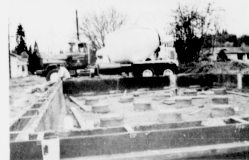
Dan and Vic Burri, cement sub-contractors, complete pouring of the Vernonia Health Center foundation. Scappoose Sand and Gravel supplied the concrete.
