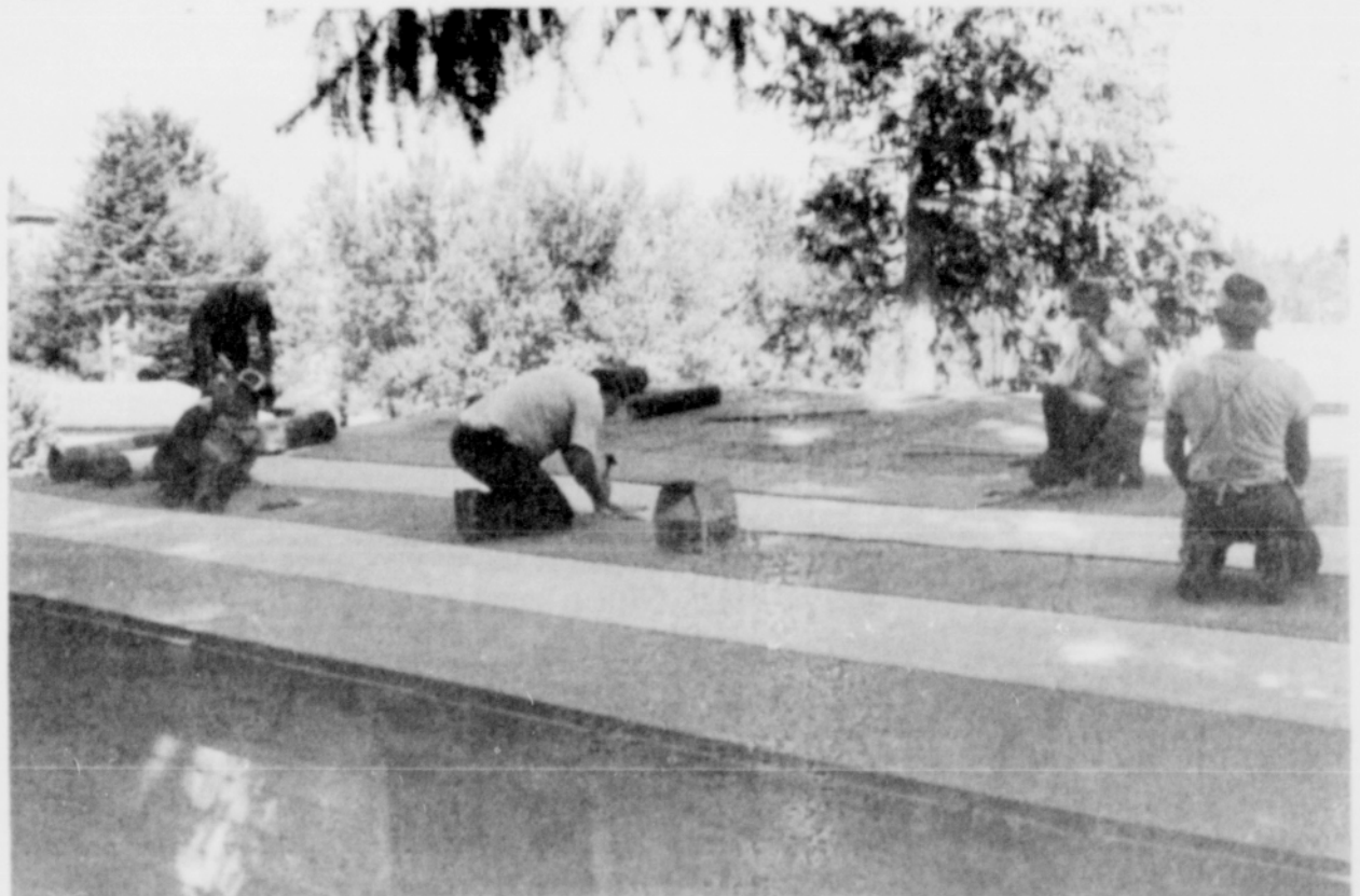
Bill Etzold, Fred Klinger, Tom Strand, Boyd Ruby and Dirk Andersen reroofed the recently purchased Chamber of Commerce building.
