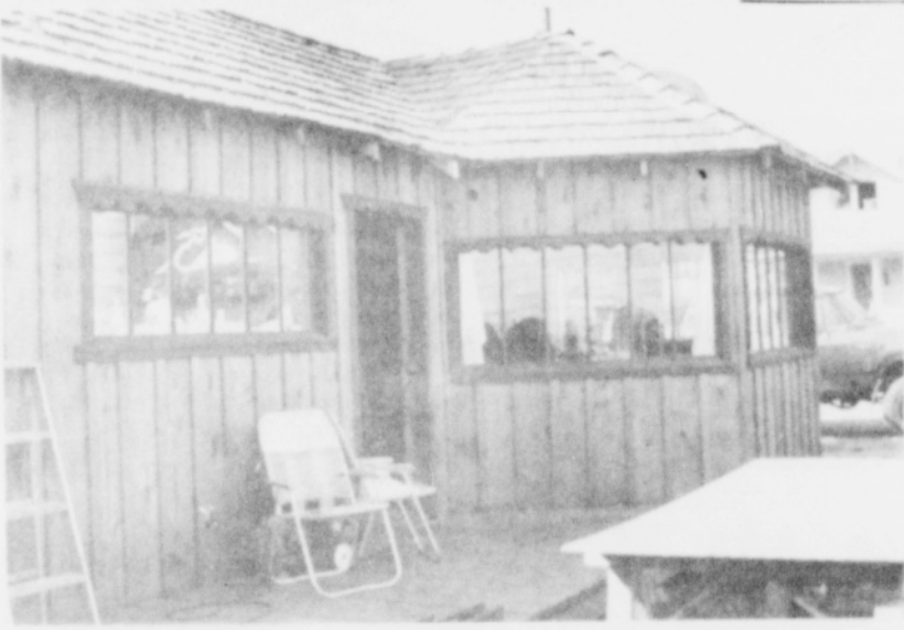
This deck on the north side of the Flour Shop will be extended to provide outdoor tables.
