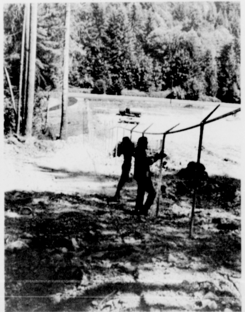
The former Arco station on Nehalem Highway south, recently purchased by Ken Smejkal has had a facelift and, in this scene, Stevens Enterprises and Jim Gardner Excavation are installing cyclone fencing on the property's perimeter. Pictured here are Scott and Lance Stevens.
