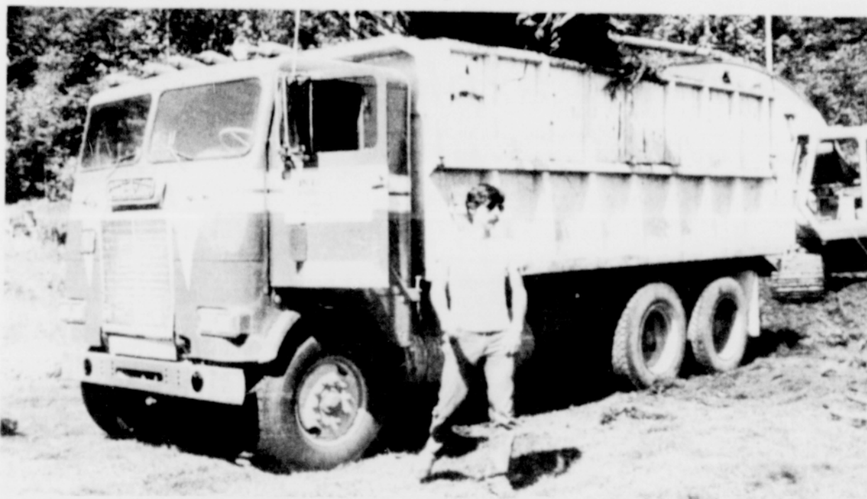
Don Leahy Demolition & Excavation truck, from Portland, is driven by volunteer Jay Koenig.
