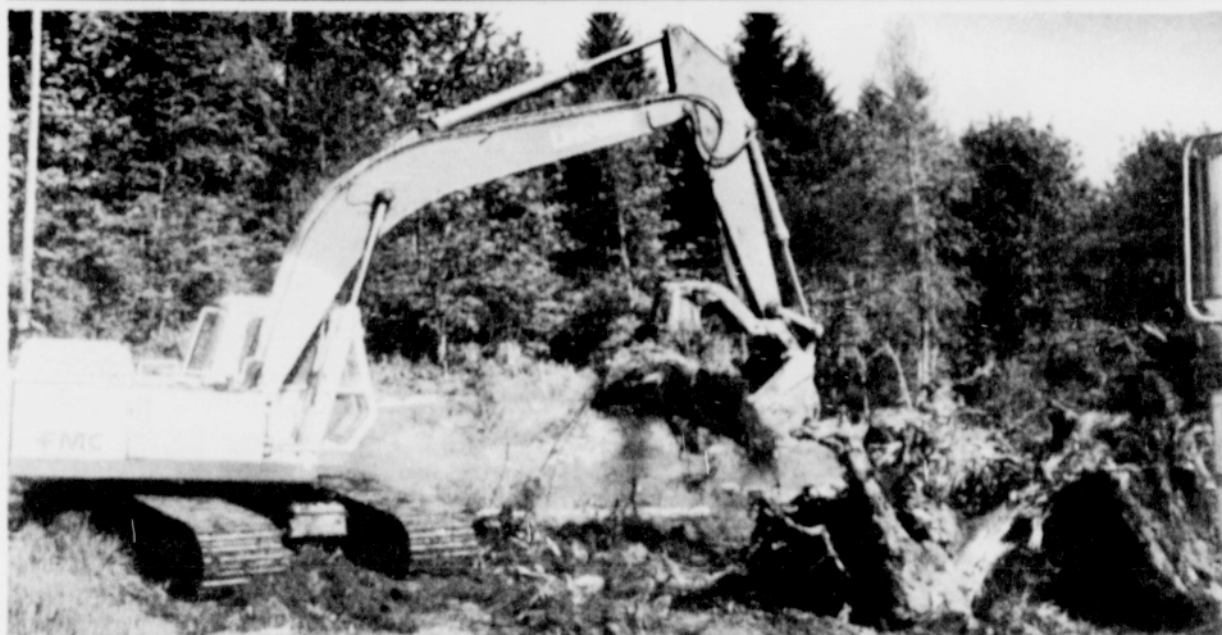
Jim Morrison, using CM Construction's shovel, uproots and loads tree stumps at the Little League ballpark.
