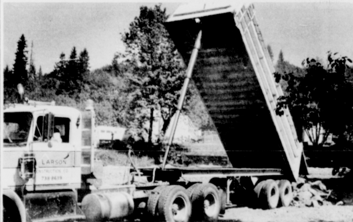
Rip rap was used to stabilize the west bank of Rock Creek.
