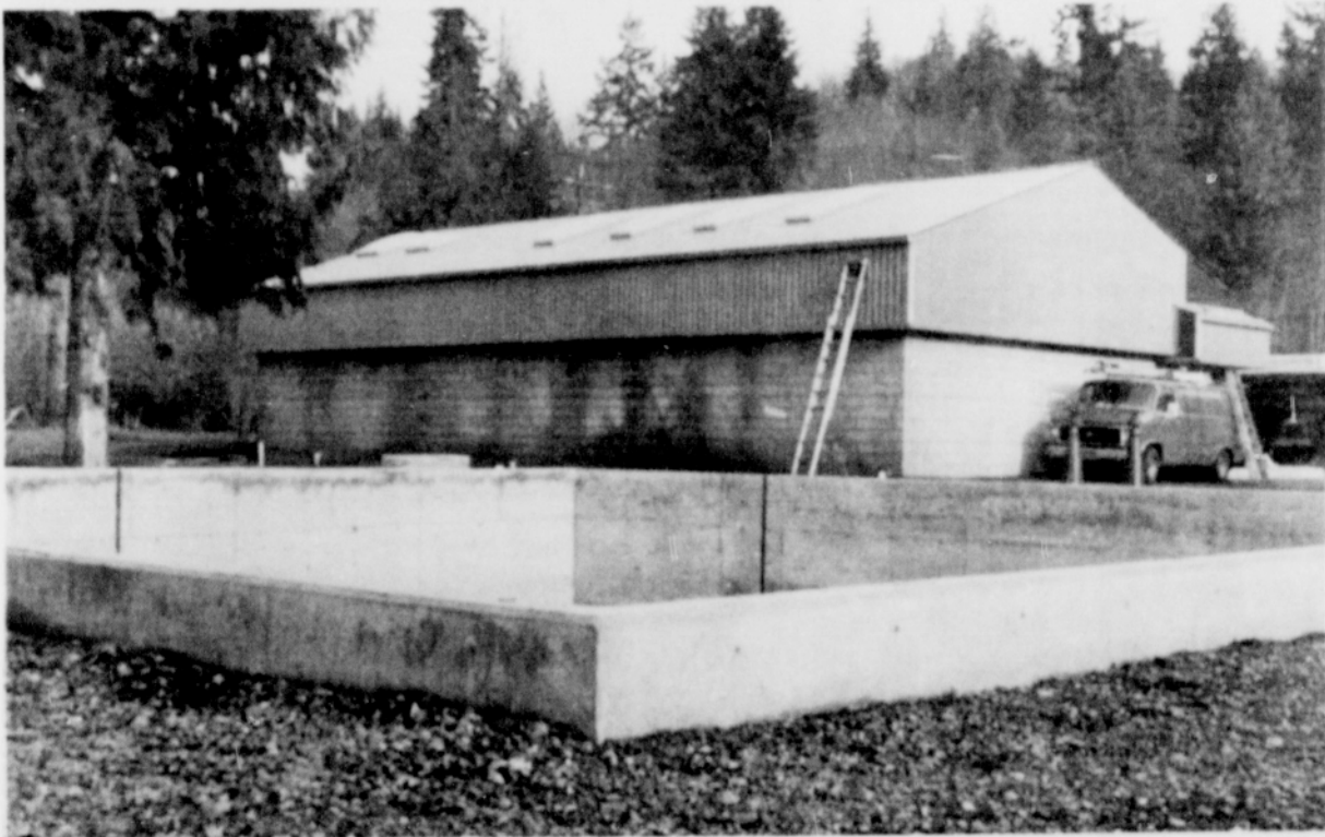
This building houses the new water treatment plant scheduled for completion in a few weeks.
