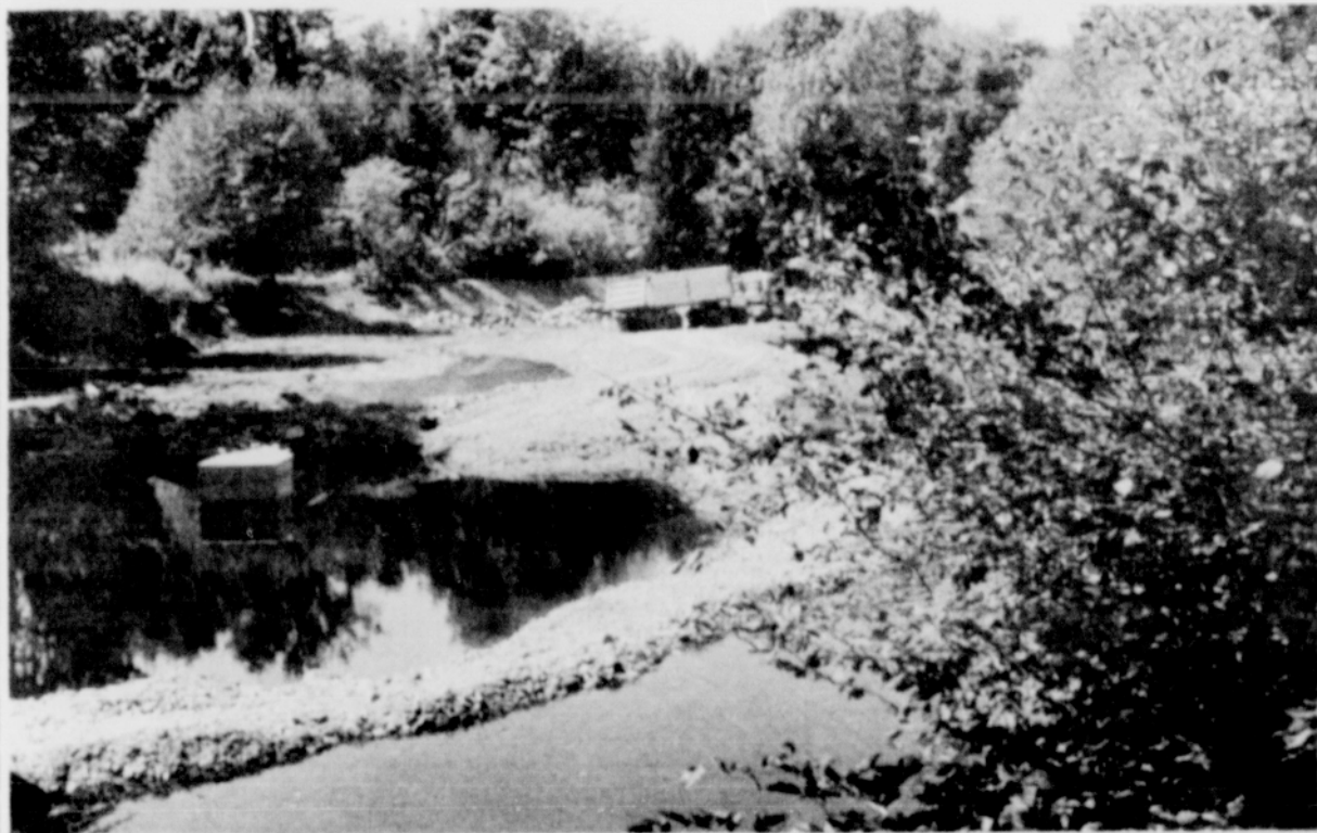
A temporary diversion of Rock Creek was necessary for construction.
