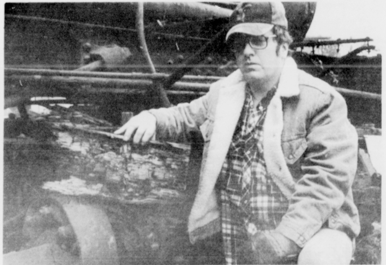
Dry rot has nearly destroyed the wood components of the Shay engine, in the beam displayed here by Tim Enyart, and in the ties that should be supporting the rails.
