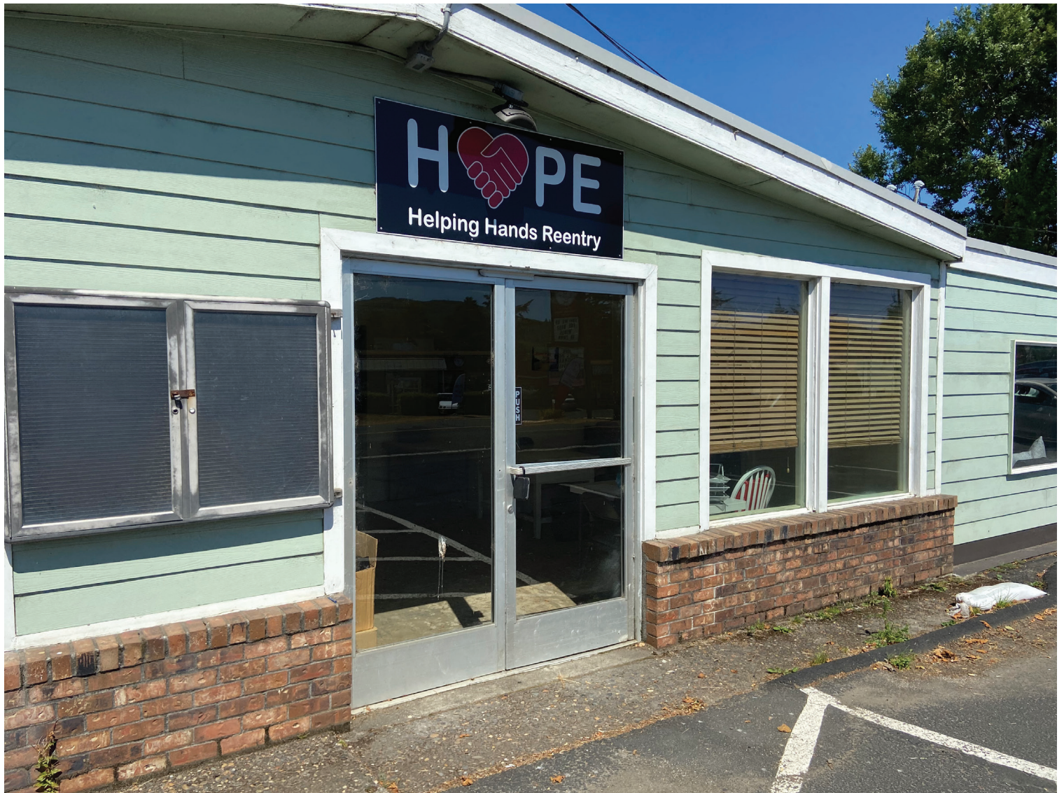
The building at 1530 N. Roosevelt serves as a seasonal warming center.
