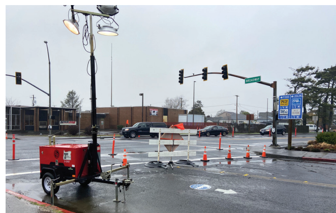
Signal work at U.S. Highway 101 and Broadway.
