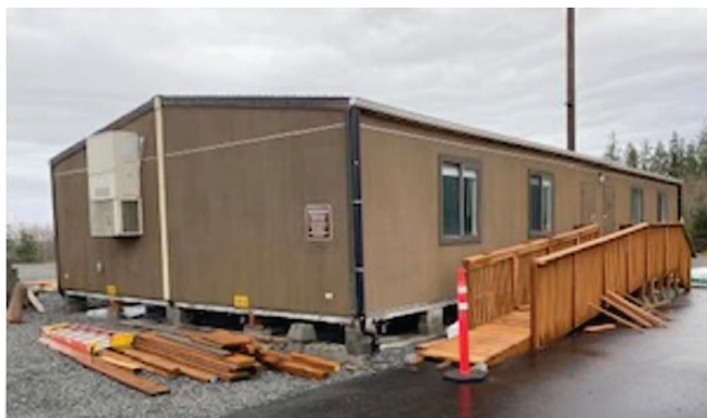
The alternate emergency operations center began as an office trailer during Seaside Civic and Convention Center renovations.
