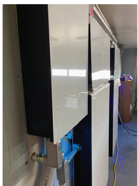
ABOVE: Ronald Bynoe in front of his South Edgewood home. LEFT: Wall panels in the basement store electricity the homeowners can sell back to the power company for credits.
