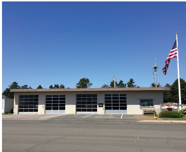
The Gearhart firehouse, built in 1958, is considered at risk in an earthquake and tsunami.
