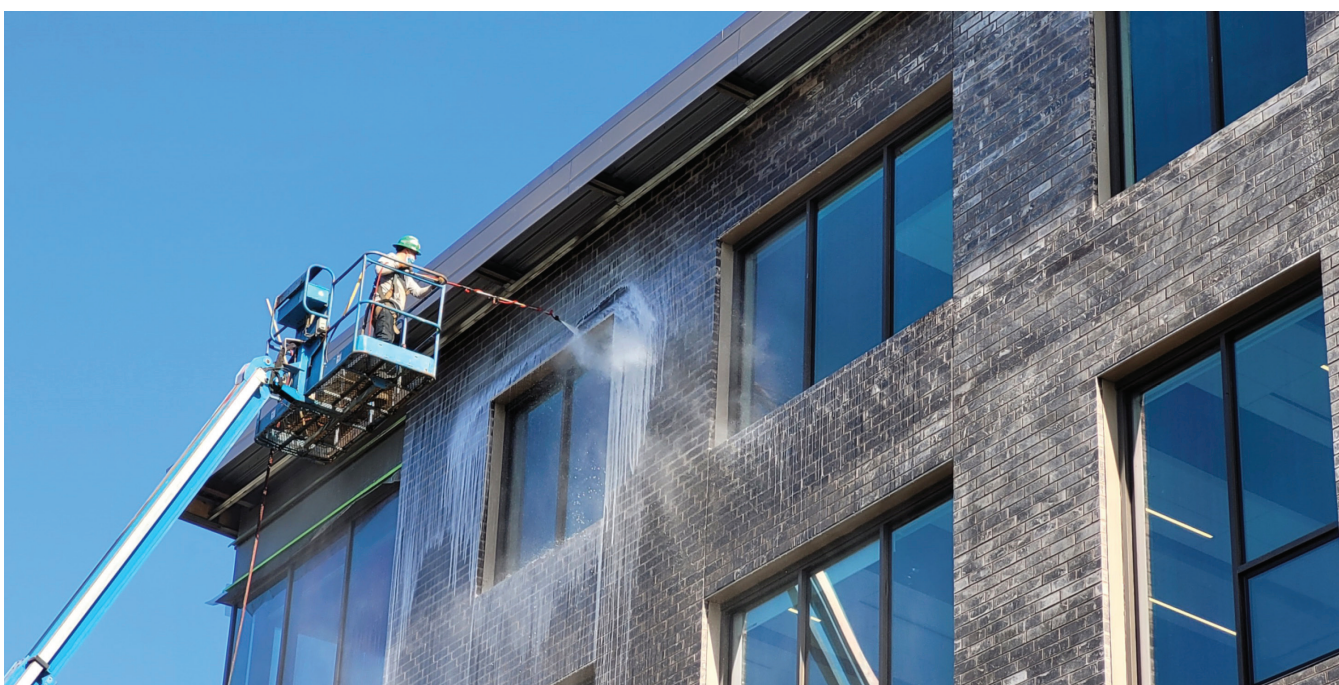
Exterior remediation at the middle and high school building.
