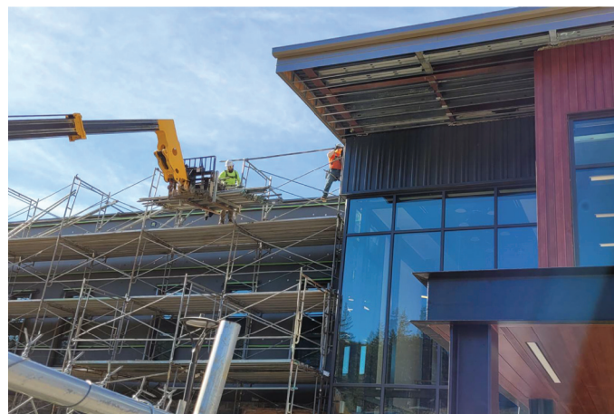
ABOVE: The athletic field at the new Seaside school campus. BELOW: Remediation on the high school and middle school building's eastern facade awaits completion.
