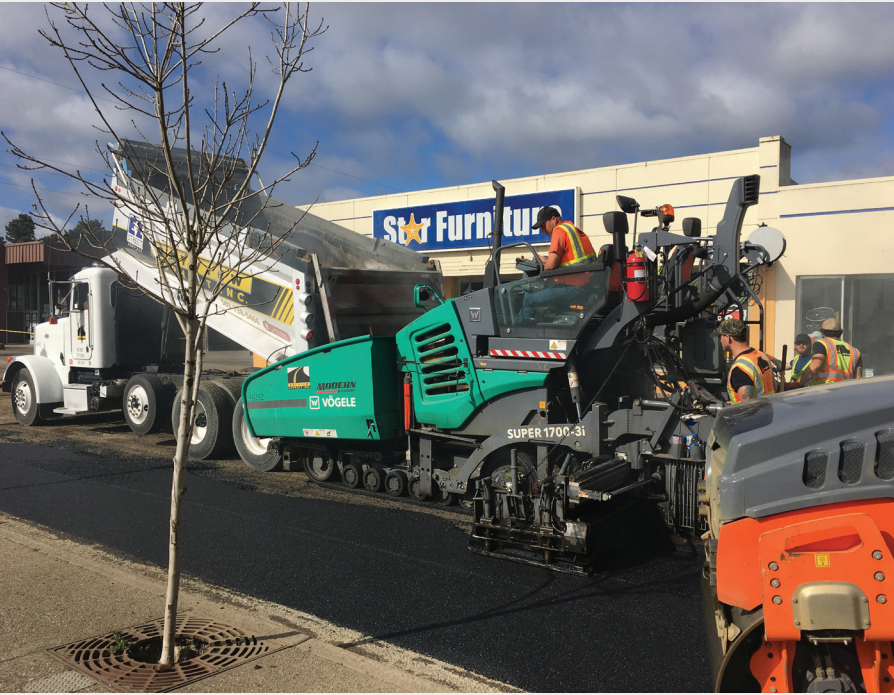
Dale McDowell/Seaside Department of Public Works Crews work on South Holladay as the Seaside Department of Public Works moved toward completion of repaving and utility upgrades.
