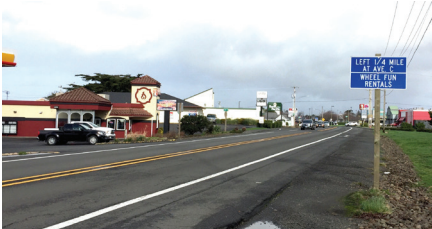
U.S. Highway 101 northbound in Seaside. The state plans work to improve the roadway, with bids starting in 2021.
