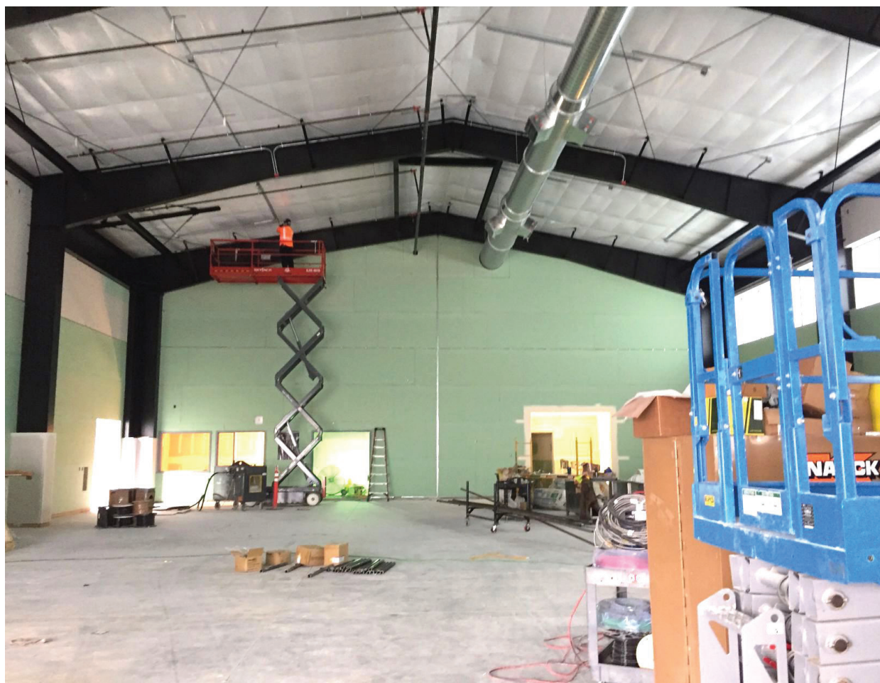
The Heights gym plans to see a wood floor installed the first week of March. The green board is impact-resistant sheet rock. The gym is scheduled to open after spring vacation.
