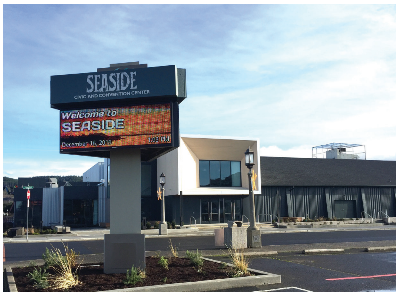
The western entrance of the Seaside Civic and Convention Center.
