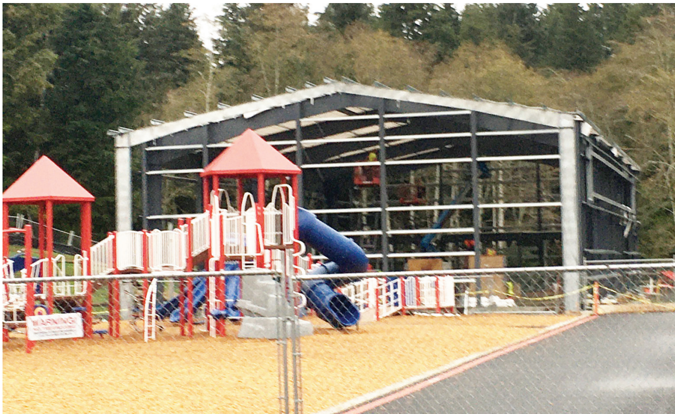
Construction of The Heights gymnasium.
