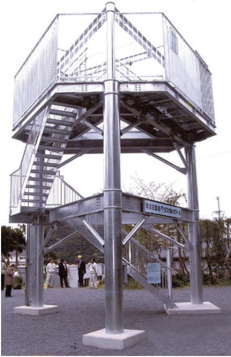
Photo of a vertical evacuation structure in Japan that was developed as a simple and economical vertical evacuation option.
