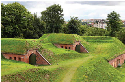
Portland Urban Architecture Research Lab Berm in Warrenton, built on privately owned land.
