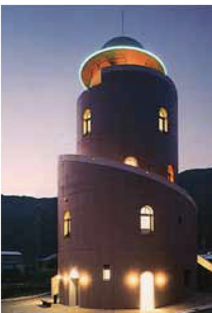
Portland Urban Architecture Research Lab Founded on a 4-meter deep layer of sand and gravel, the tower in Nishiki, Japan, is supported on concrete piles extending 6m below grade. It was designed to withstand the impact of a 10-ton ship at a velocity of 10m/sec.
