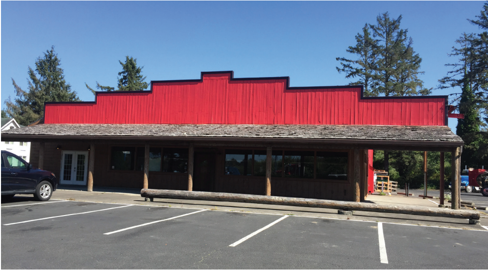
The former site of Bigfoot’s will be used storage space for Seaside Brewing Co.
