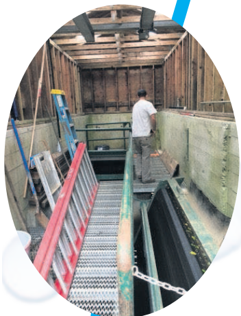
Kevin Nagle inside the diversion building.
