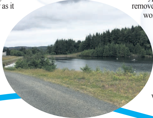
Seaside's reservoir at Peterson Point.
