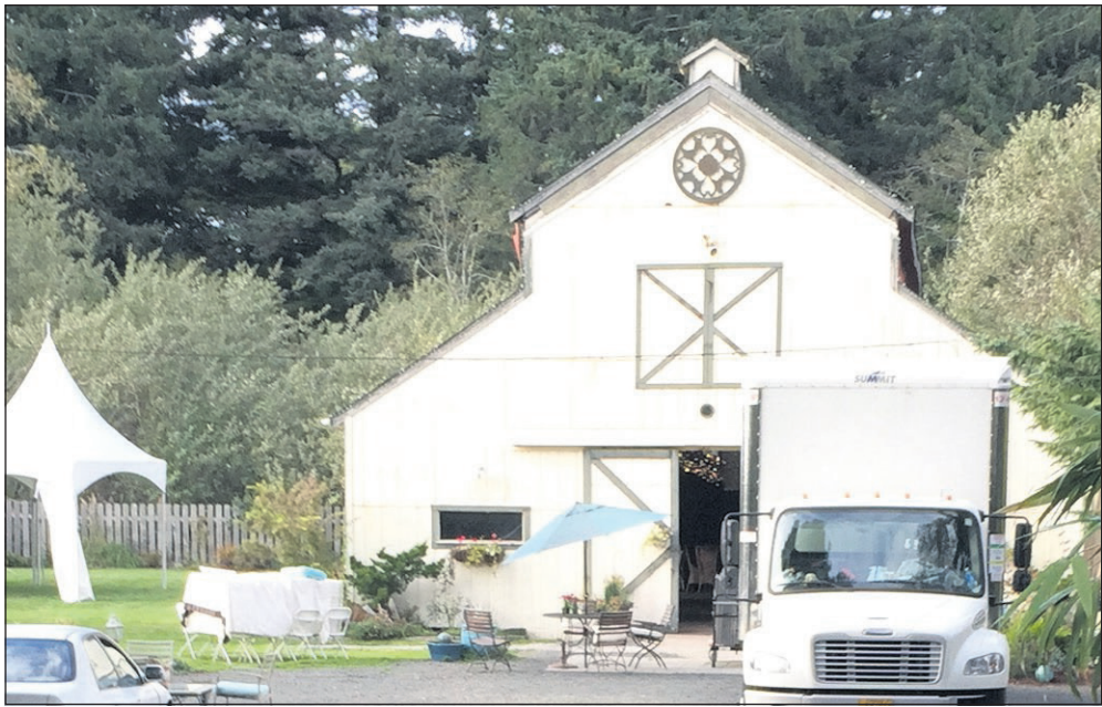
The Neacoxie Barn was fined in 2015 for its use as a party venue without a certificate of occupancy.
