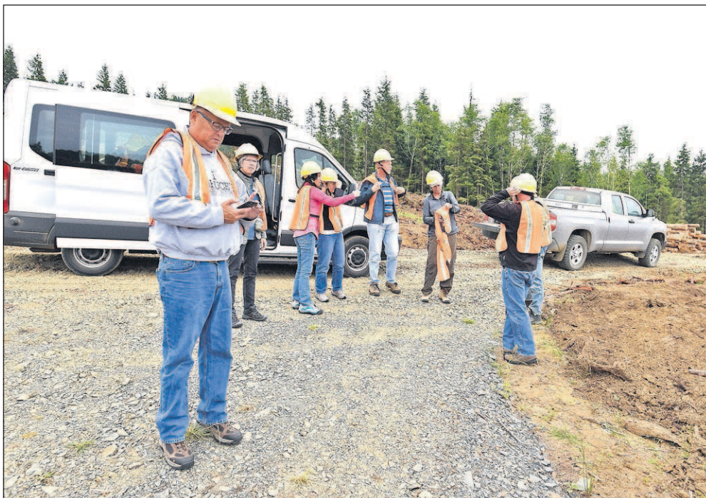
Seaside School District board members toured the school construction site during logging operations.
