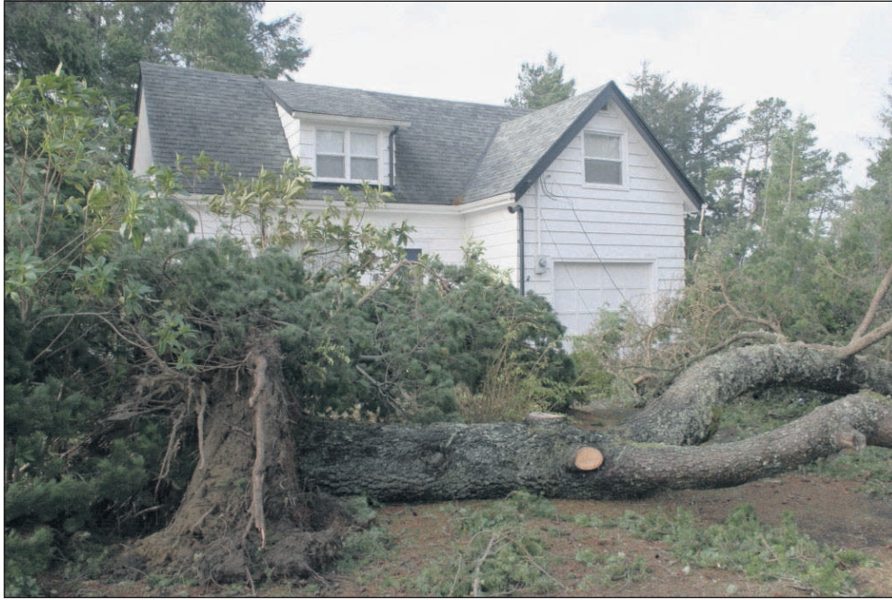
Trees down in front of a Seaside home in the wake of the storm.
